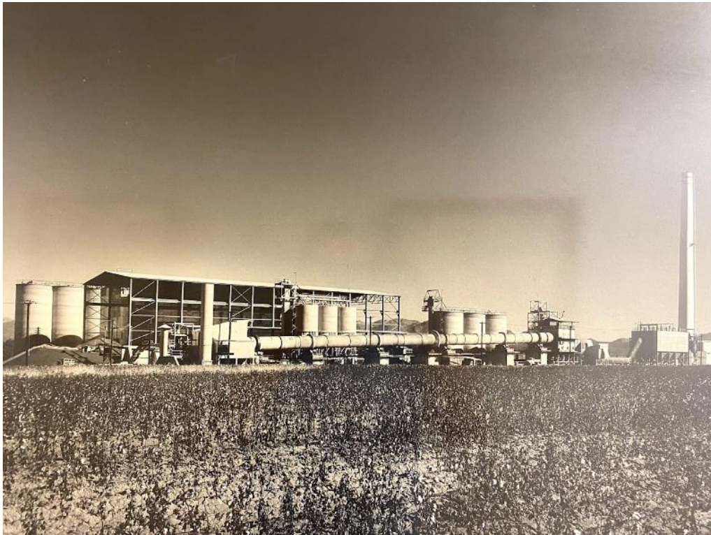
Rillito Cement Plant First Kiln installed 1949
