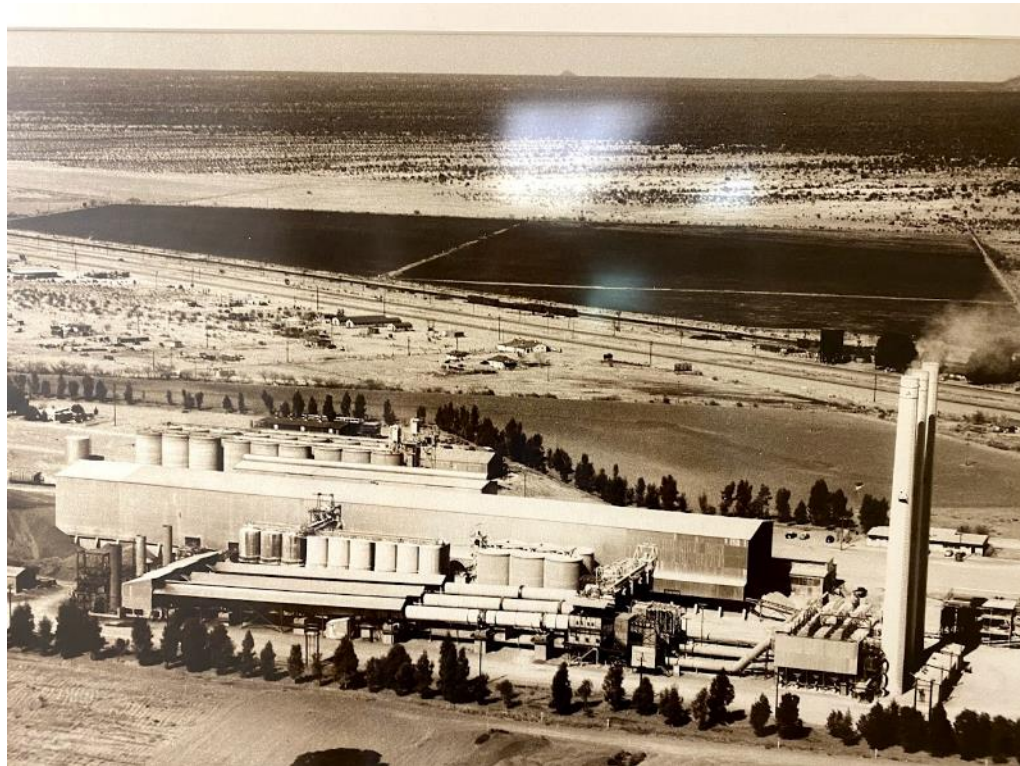
Rillito Cement Plant Third Kiln installed 1955
