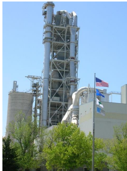
Figure 1. ENERGY STAR Certified Cement Plant
