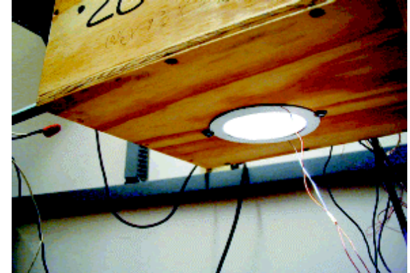
Photo 3. Temperatures of combustible building materials may not exceed 90°C
