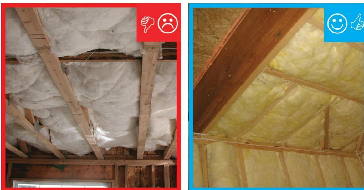
**Figure 1 – Improper Installation versus Grade I Quality**
