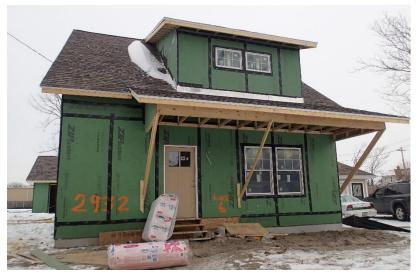
A home is considered "dried in" when the roof is completed; at this time the insulation can be added. The above home is in the process of being insulated.
