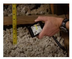
Figure 1. Measuring the depth of attic insulation.
