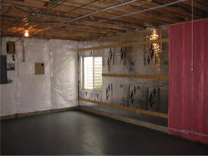
Figure 10. Foil-faced polyiso foam is held in place along the interior of a basement wall with nails or screws through the furring strips. Seams are sealed with foil tape and all edges are sealed with caulk or foam. (Source: [Measure Guideline: Basement Insulation Basics](#)).
