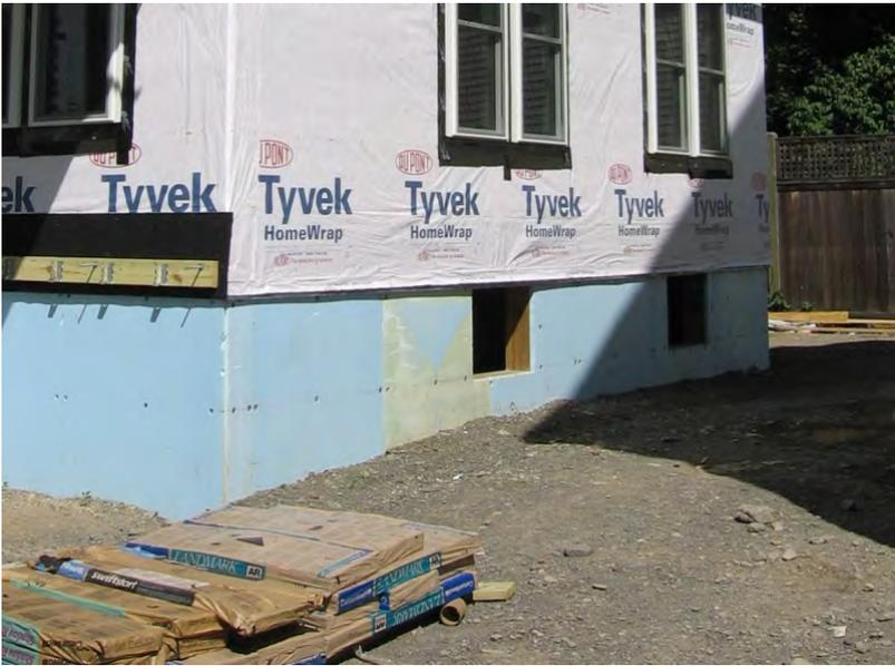
Figure 3. Exterior XPS basement insulation is correctly installed to completely cover the foundation wall.
