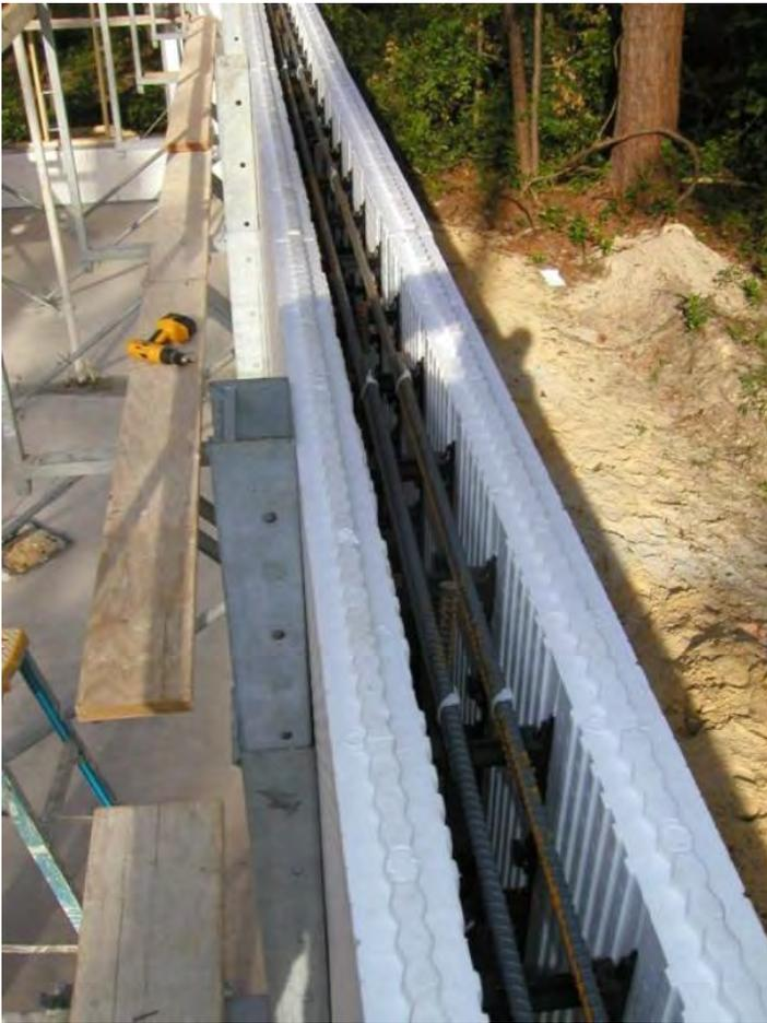
Figure 7. ICF bricks are stacked to form hollow walls that are reinforced with steel rebar before the concrete is poured in. (Source: [Measure Guideline: Basement Insulation Basics](#)).
