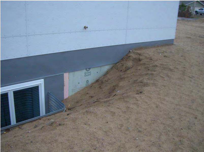
Figure 4. Rolled fiberglass sheets are installed to protect exterior XPS at and above grade.
