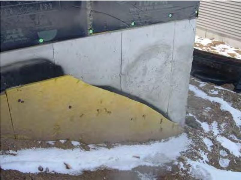
**Figure 1.** Exterior fiberglass insulation on this new home was (incorrectly) cut to terminate below-grade after backfill, which will expose the above-grade portions of the foundation wall to cold temperatures. (Source: [Measure Guideline: Basement Insulation Basics](#))
