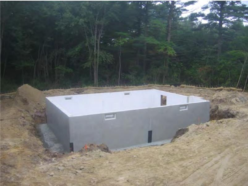
Figure 9. A precast insulated concrete panel foundation is set in place on a base of crushed rock. (Source: [Measure Guideline: Basement Insulation Basics](#)).
