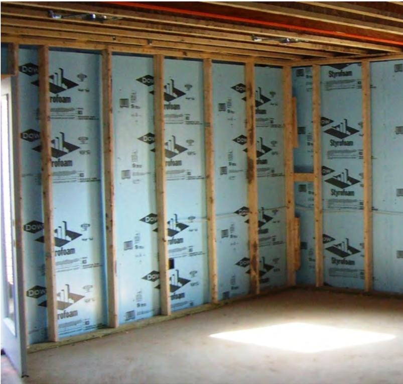
Figure 12. XPS is installed along basement walls before constructing a framed wall. (Source: [Measure Guideline: Basement Insulation Basics](#)).
