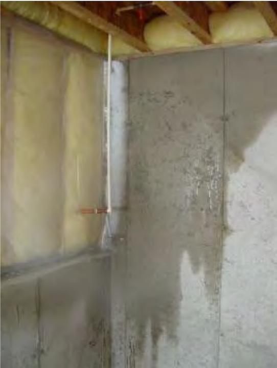
**Figure 2.** Because the above-grade portions of the wall lack exterior insulation, condensation and even ice form during cold winter conditions. (Source: [Measure Guideline: Basement Insulation Basics](#)).
