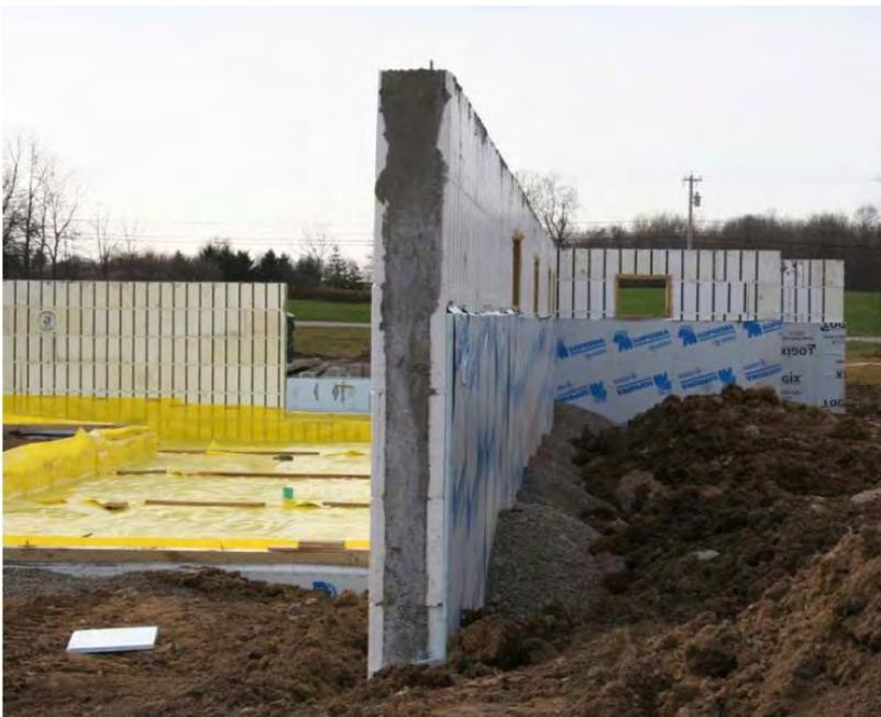
Figure 8. ICFs can be used below and above grade to construct the entire wall. (Source: [Measure Guideline: Basement Insulation Basics](#)).
