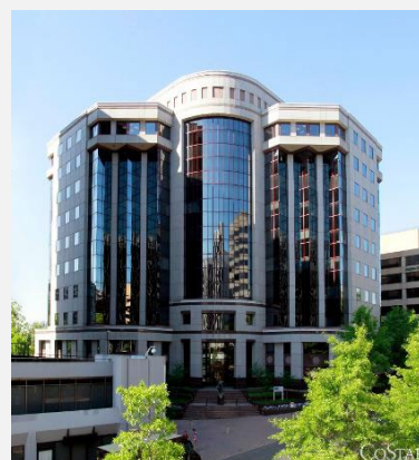
1530 Wilson Boulevard, Arlington, VA. First ENERGY STAR certified in 2007.
