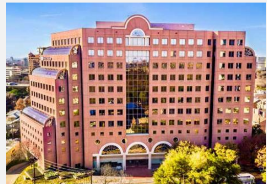
3131 McKinney, Dallas TX. First ENERGY STAR certified in 2008.
