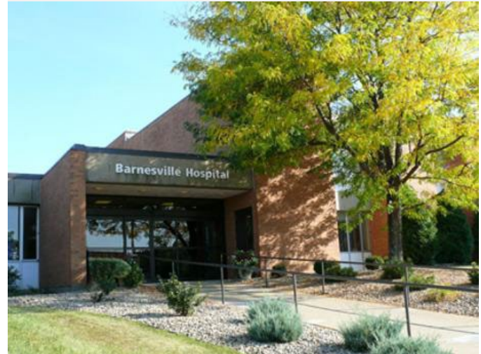
Barnesville Hospital, Barnesville, OH. ENERGY STAR certified since 2016.
