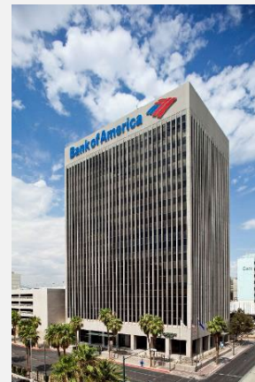
Bank of America Plaza, Las Vegas, NV. First ENERGY STAR certified in 2019.
