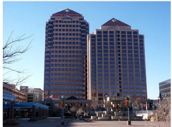
Albuquerque Place Office Investment LLC, Albuquerque, NM. First ENERGY STAR certified in 2013.
