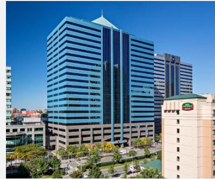
545 Washington Blvd, Jersey City, NJ. First ENERGY STAR certified in 2020.
