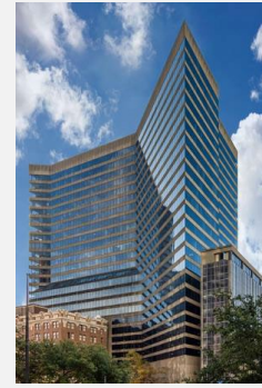
Poydras Center, New Orleans, LA. First ENERGY STAR certified in 2002.
