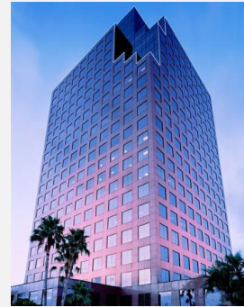
110 Tower, Ft. Lauderdale, FL. First ENERGY STAR certified in 2010.
