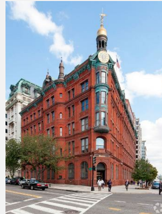
1445 NY Avenue, Washington, DC. First ENERGY STAR certified in 2010.
