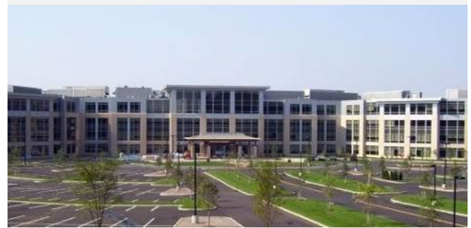
Voya Windsor Facility, Windsor CT. First ENERGY STAR certified in 2009.
