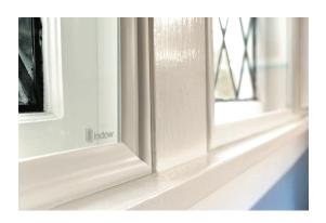
be very easy to install and remove they can be constructed as a monolithic panel. If an occupant wishes to operate the primary fenestration they can easily and very quickly remove the interior storm window entirely. The option to create a monolithic panel that covers the entire inside surface of the window frame means that interior storm windows can be very airtight.
