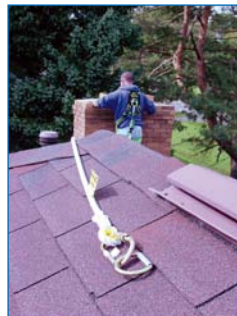
Figure 7: Roof anchor should be installed on a roof subsurface or vertical wall.
