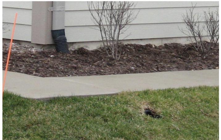
*The drain slopes away from the foundation and terminates at the proper distance.*
