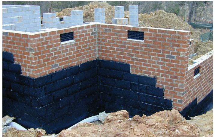
*The below-grade concrete walls have damp-proof coating.*
