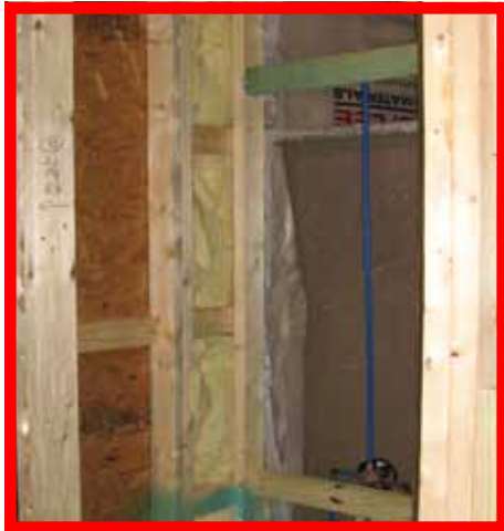
A. No backing installed behind shower enclosure.
