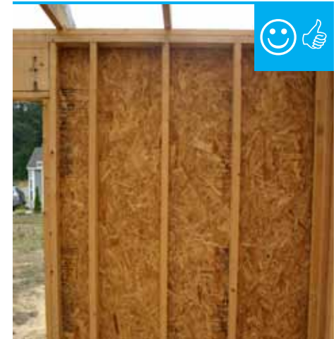
Building materials were kept dry and free of mold.
