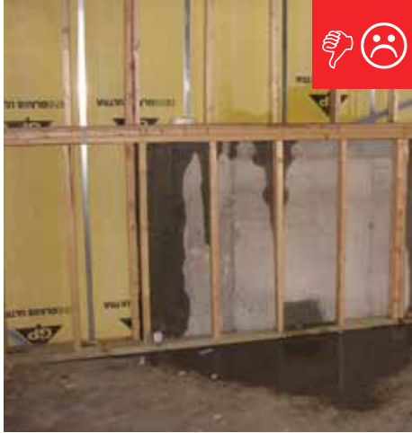
A. Untreated lumber has been used on a below-grade wall against masonry.
