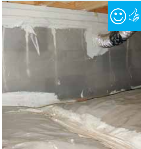
There is polyethylene sheeting installed and sealed in the crawlspace.
