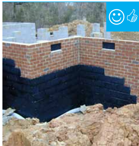
The below-grade concrete walls have damp-proof coating.
