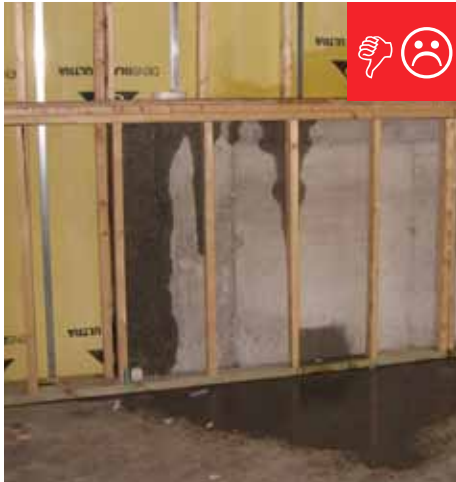
A. The below-grade concrete does not have the correct mixture to be impermeable to moisture.
