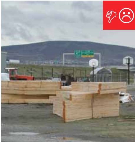
A. Building materials are being stored outdoors with no protection from weather.
