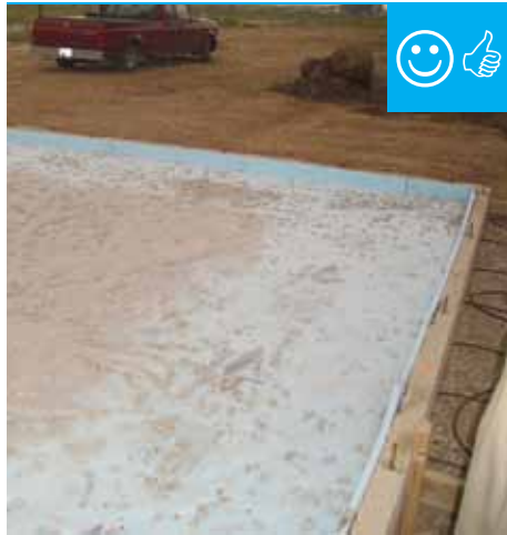
There is polyethylene sheeting installed to provide a capillary break between the ground and slab.
