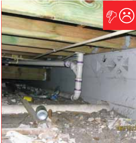
B. There is no polyethylene sheeting installed in the crawlspace.
