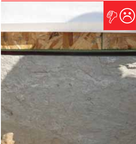
A. There is not a weep screed installed at the bottom of the stucco wall.
