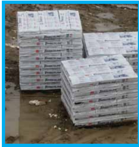
Shingles kept wrapped and on pallets to prevent from getting wet.
