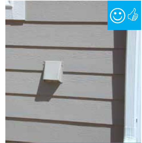
Ventilation inlet is appropriately located above grade.
