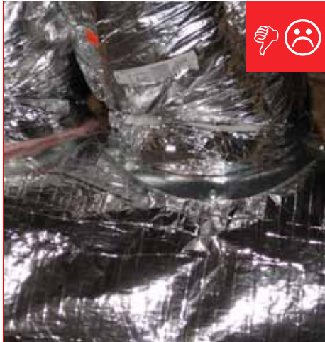
A. Trunk to duct connections are only mechanically fastened and not sealed.
