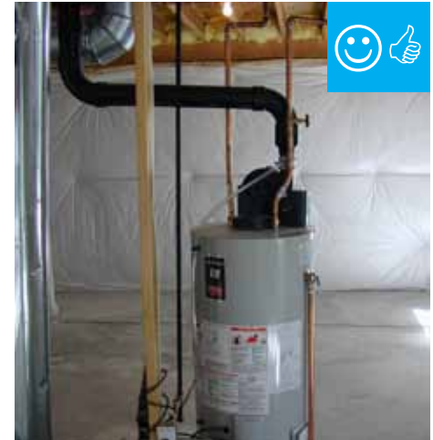
Power vented water heater installed.
