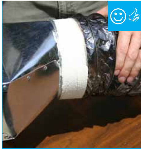
Mechanically fastened and sealed.
