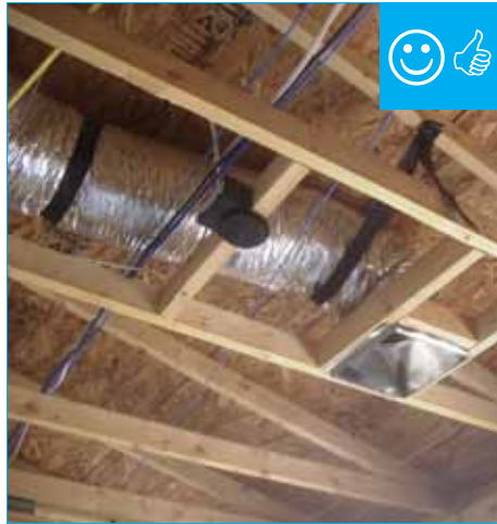
Duct is run straight and supported properly.
