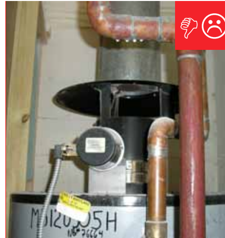
A. Naturally drafted water heater installed. Requires combustion safety testing.
