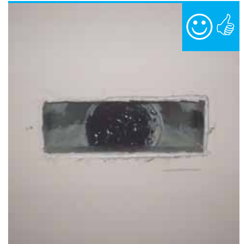
Boot to drywall connection sealed.
