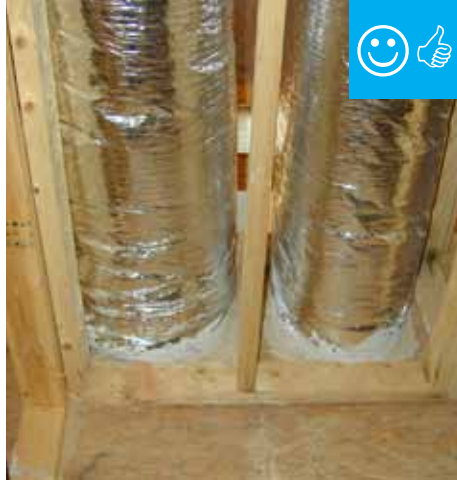
Framing allowed duct work to be properly installed without compression.
