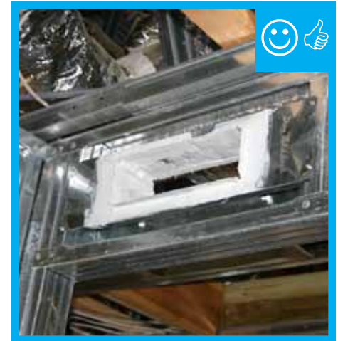
Transfer grill sealed with mastic.
