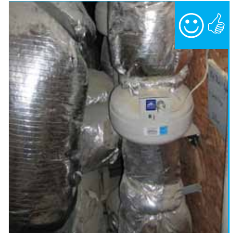
In line exhaust ventilation installed.
