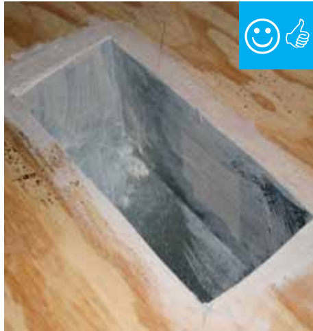
Boot to floor connection sealed.
