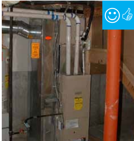
Direct vent appliance installed.
