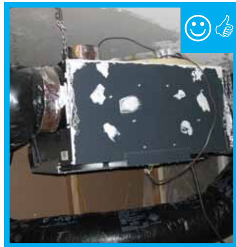
Properly installed ERV/HRV.
