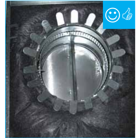
Mechanical damper installed.
