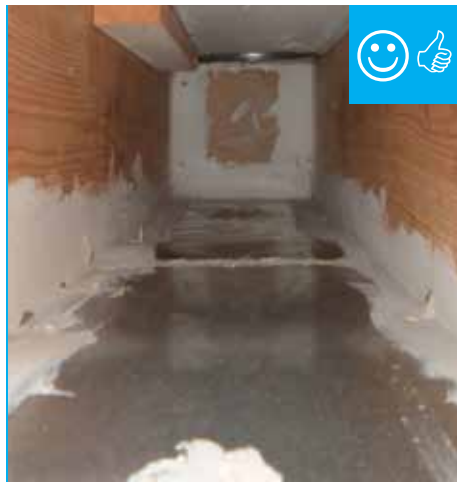
Cavity has been air sealed with mastic.
