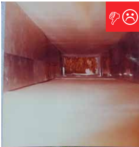
D. Cavity was not air sealed.
