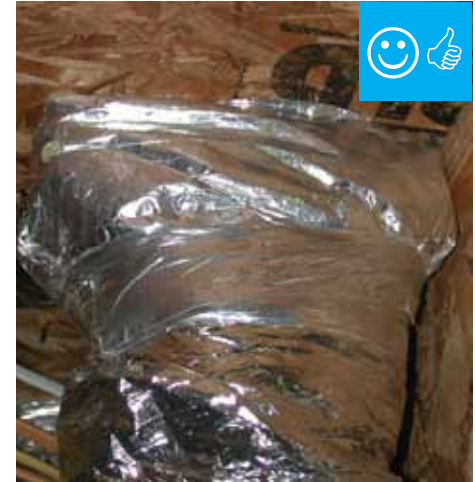
Duct insulation is installed over boot.
