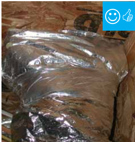
Duct insulation is installed over boot.
