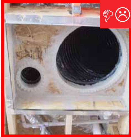
A. Ventilation tied into the return without a mechanical damper.
