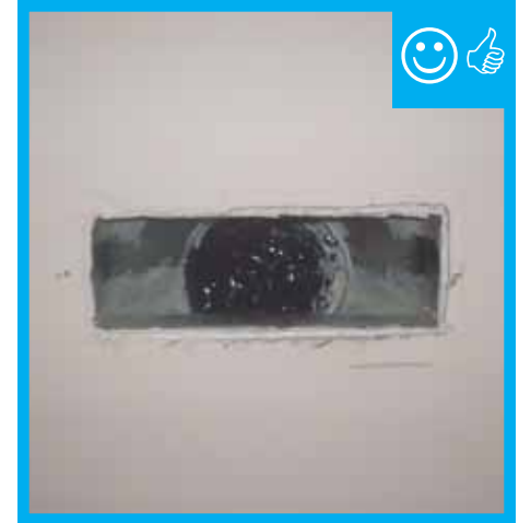
Boot to drywall connection sealed.
