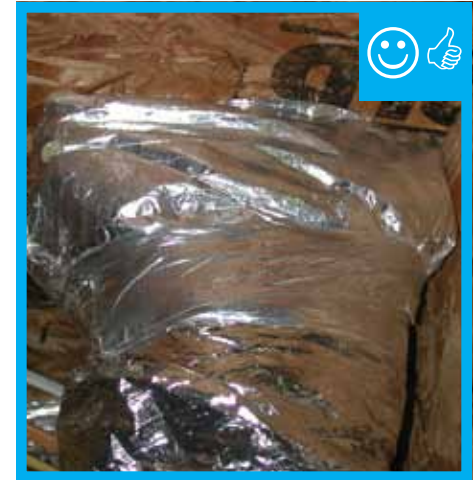
Duct insulation is installed over boot.
