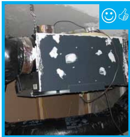
Properly installed ERV/HRV.
