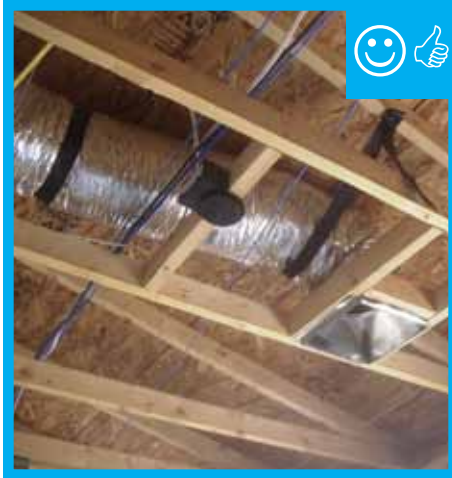
Duct is run straight and supported properly.
