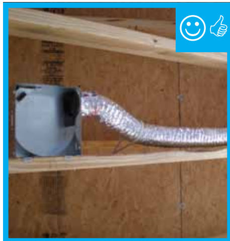
Fan housing was oriented in the correct direction to allow proper exhaust duct installation.
