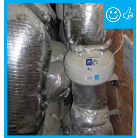
In line exhaust ventilation installed.
