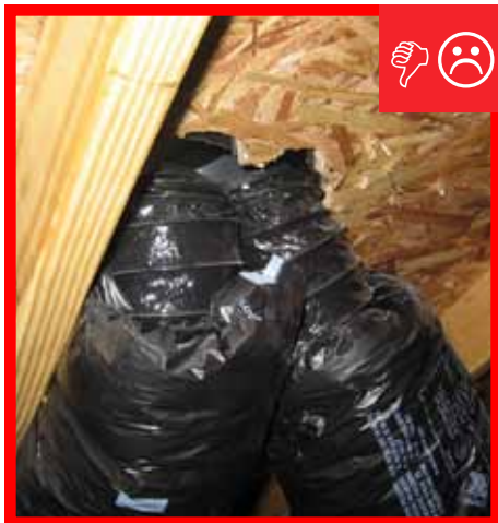
C. Fans from separate dwellings exhausted together without back-draft dampers and not sealed.
