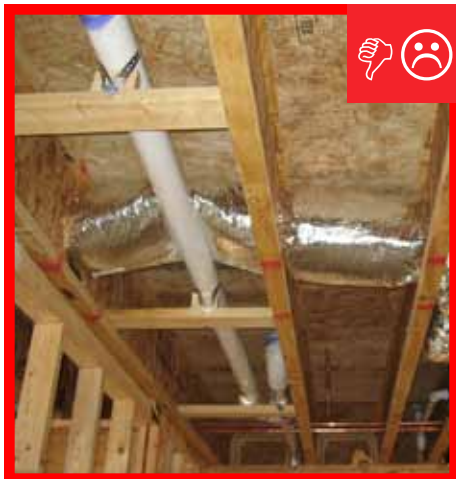
A. Duct is compressed.
