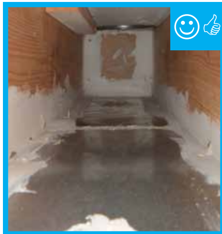
Cavity has been air sealed with mastic.
