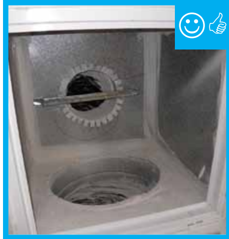
Ventilation tied into the return with a mechanical damper.
