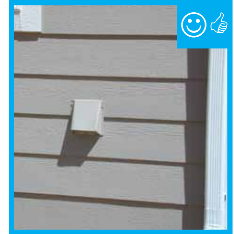
Ventilation inlet is appropriately located above grade.
