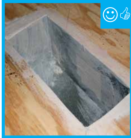
Boot to floor connection sealed.
