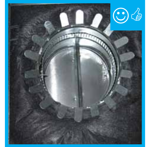
Mechanical damper installed.
