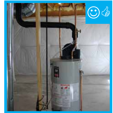
Power vented water heater installed.
