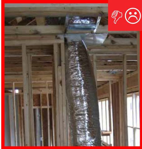
A. Duct is compressed.
