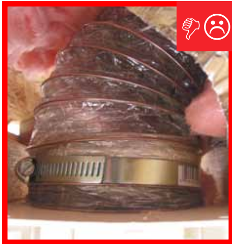
A. Connection in place but not sealed.
