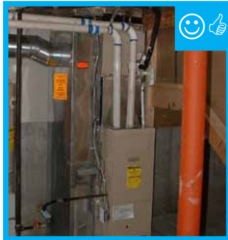
Direct vent appliance installed.
