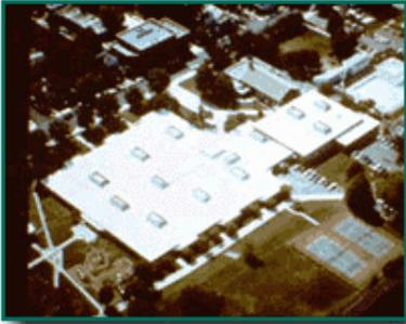
*An old, failing roof was replaced with a highly reflective, insulated, single-ply membrane roofing system. The new roof resulted in increased comfort and substantial savings with no additional cost for the higher performance.*
